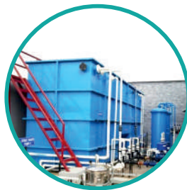
SEWAGE TREATMENT PLANT
